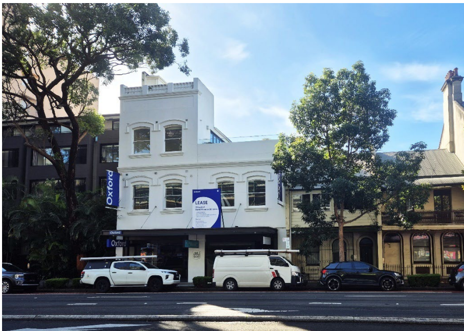
16 40-42 Flinders Street viewed from the south-west.
