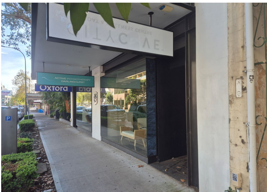
18 Shopfronts at 40-42 Flinders Street.
