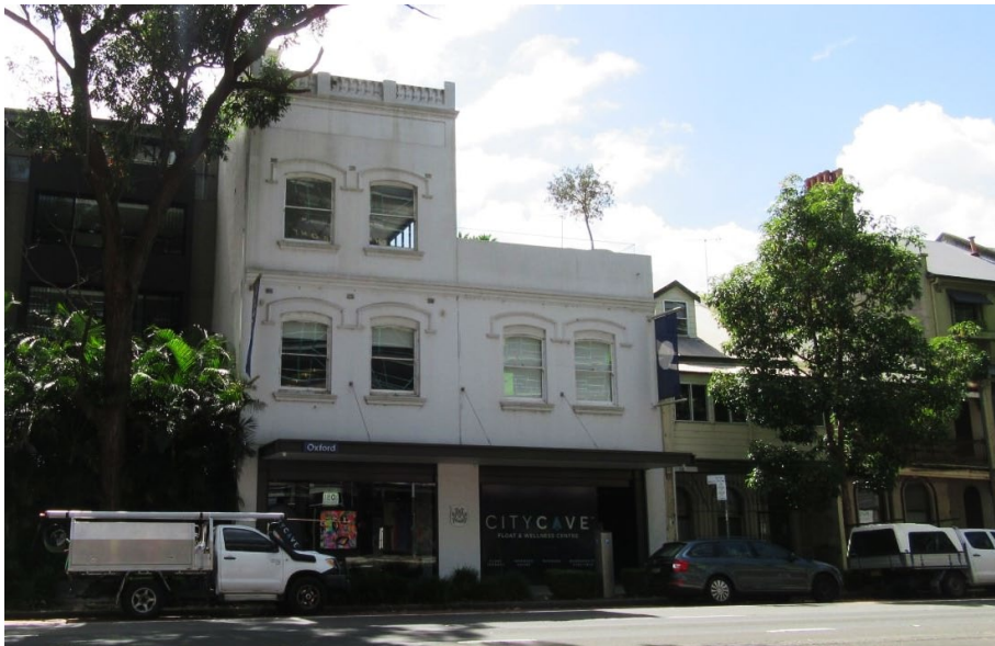
17 Façade of 40-42 Flinders Street, taken in 2023.
